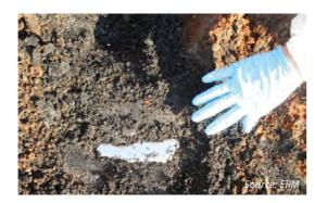
Following investigation, any environmental boreholes must be properly backfilled with expandable grout (e.g. bentonite) to avoid creating preferential pathways,
