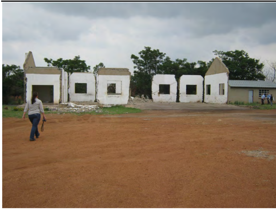
Photo 6 Facing South on the Proposed Site
