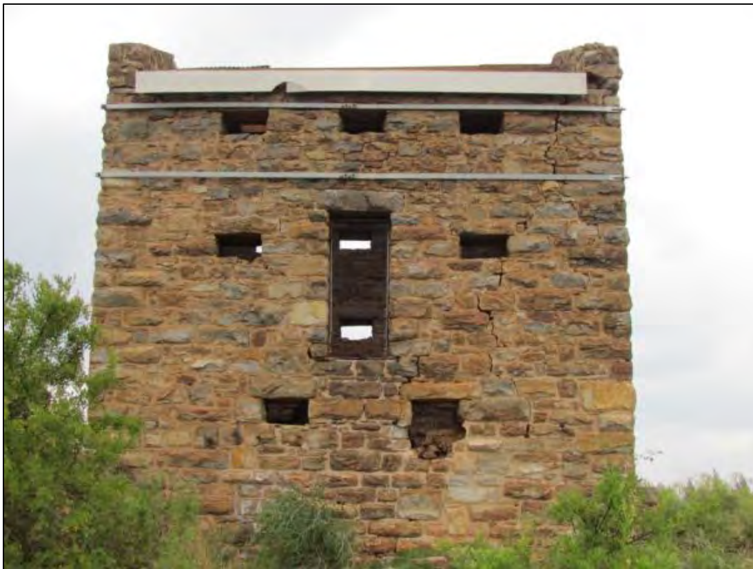
Figure 6-1: Witkop Blockhouse (Photograph by N Higgitt, 2013)
