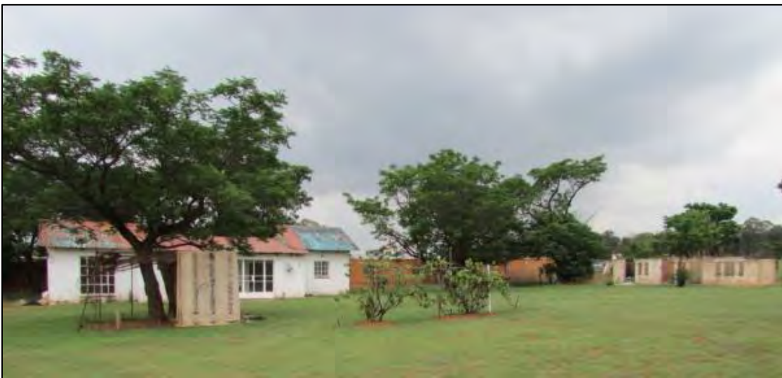
Figure 6-11: Adjacent outbuildings on Stand 89. (Photograph by N Higgitt, 2013)
