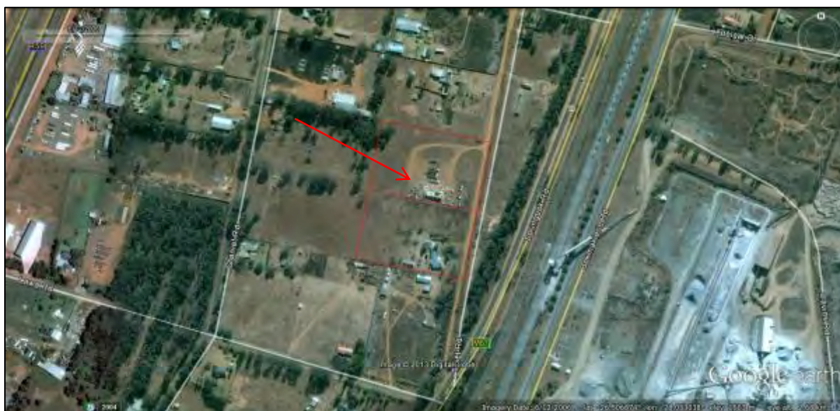
Figure 6-7: Google Earth aerial image from 6/12/2006 showing the construction of the house on Stand 88.
