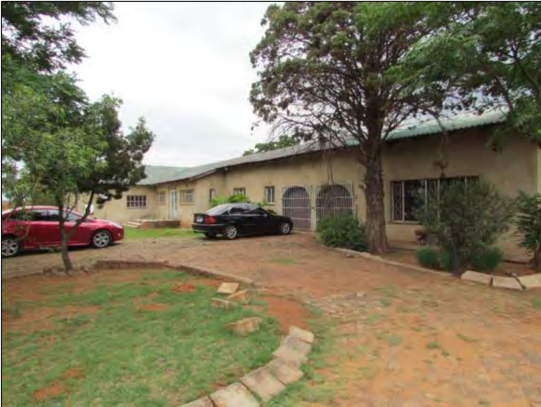
Figure 6-10: Main house on Stand 89 built in approximately 1980. (Photograph by N Higgitt, 2013)
