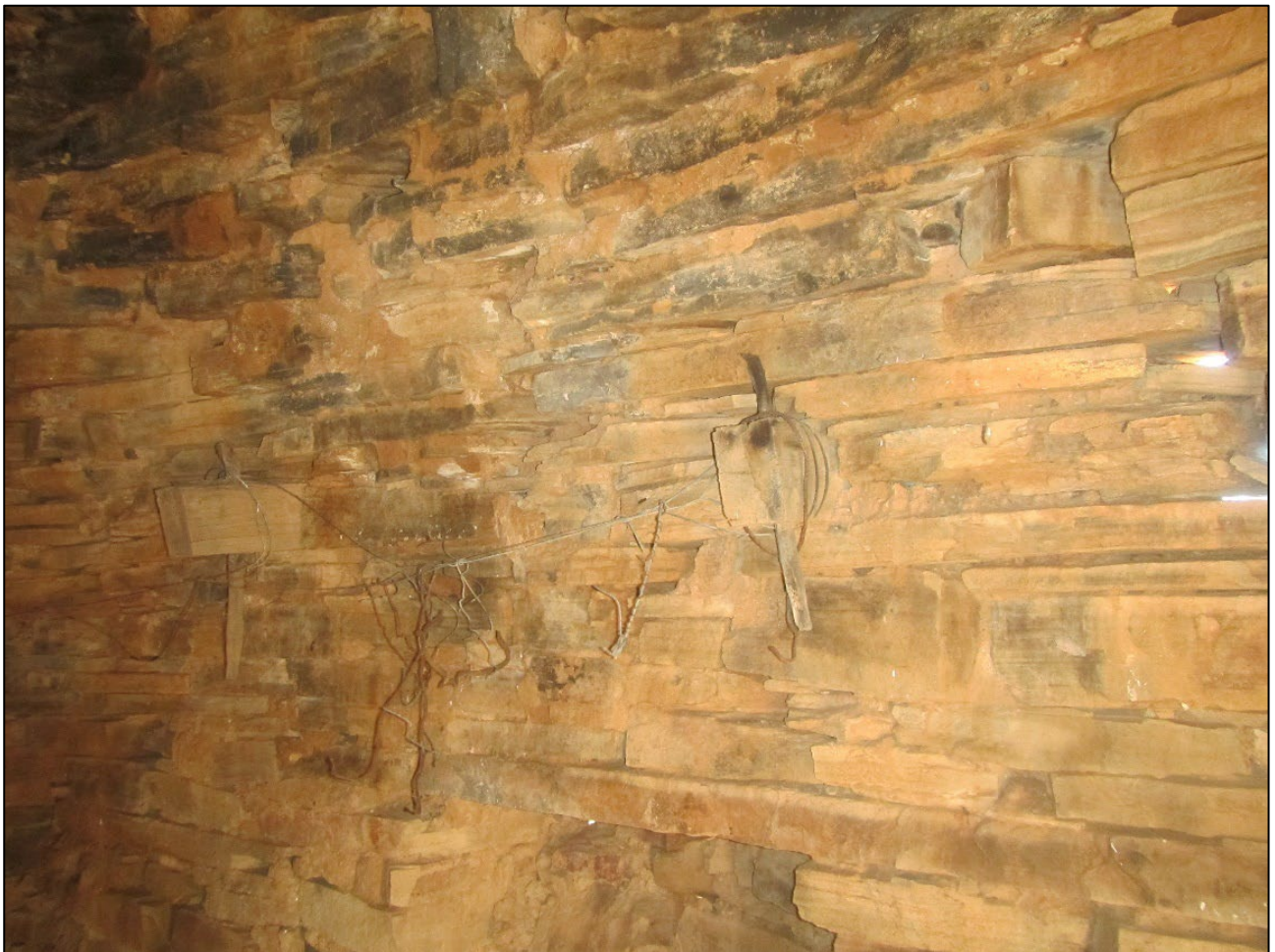
Figure 24: Internal features of the corbelled building at waypoint 1270. Two pierced wooden blocks with pegs through them are visible in the wall above the lintel of the now closed up northern door. Some wire has been fastened to the wooden blocks.
