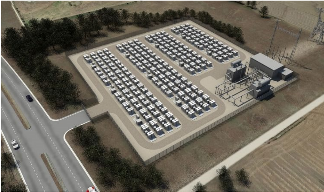
Plate 8-6: SolarCity's Tesla Battery Storage facility, Hawaii.
