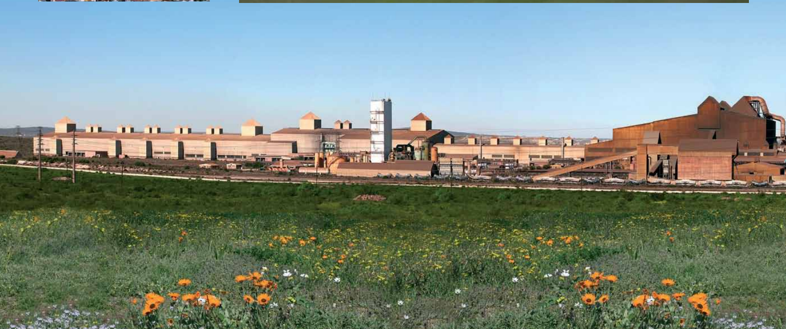
Example of a gas-fired power plant
