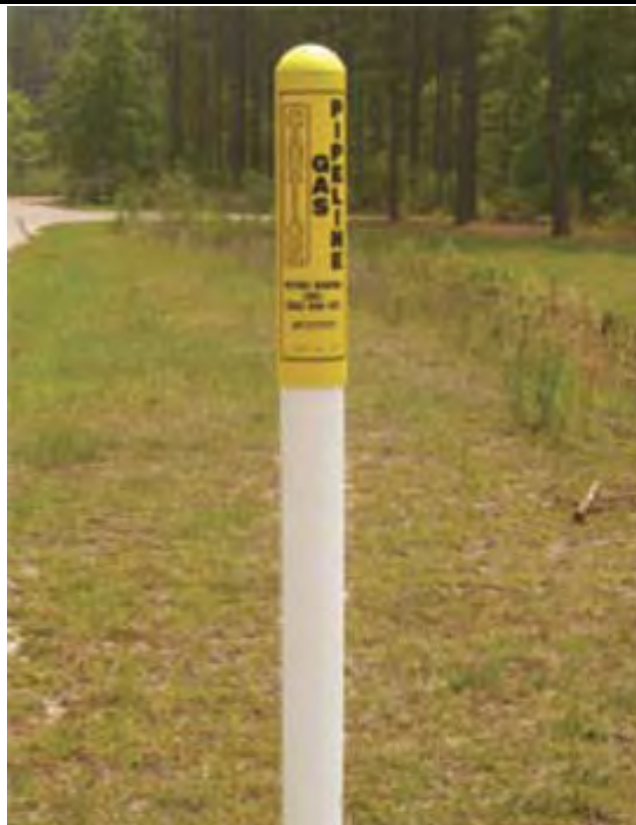
Figure 2.6 Example of a marker indicating pipeline below ground
