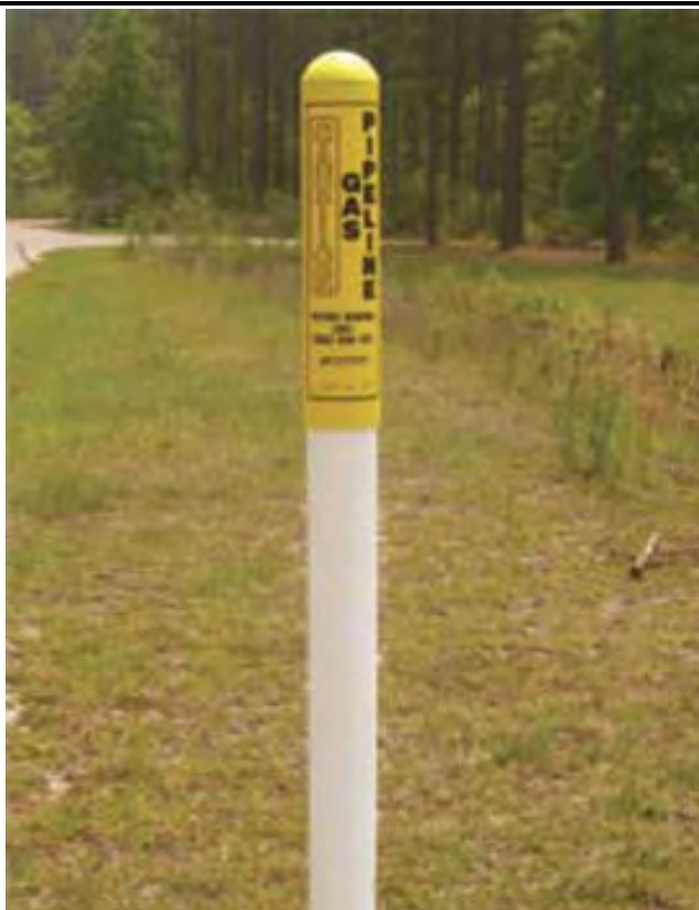
Figure 11.6 Example of a marker indicating pipeline below ground
