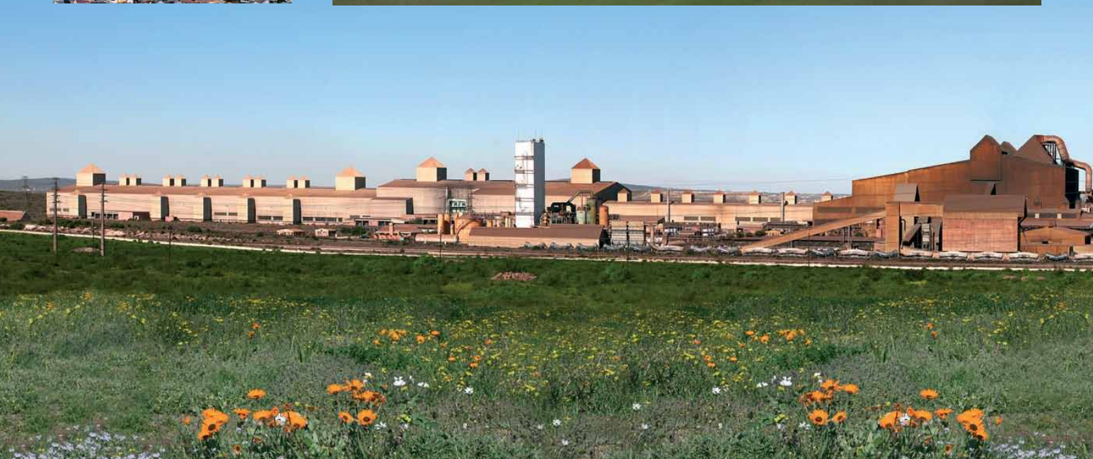
Example of a gas-fired power plant
