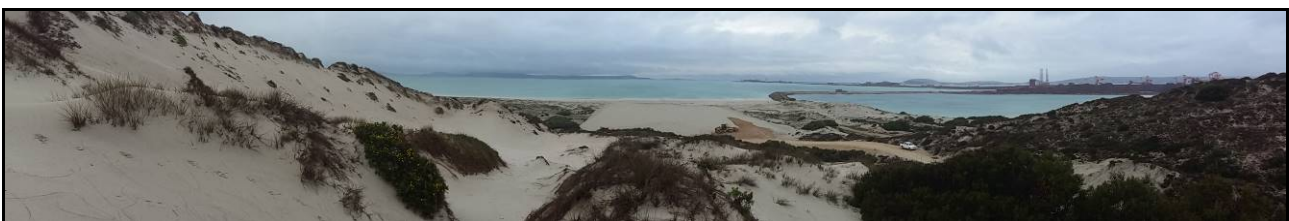
Plate 1: The pipeline comes ashore in an area which has already been extensively transformed.
