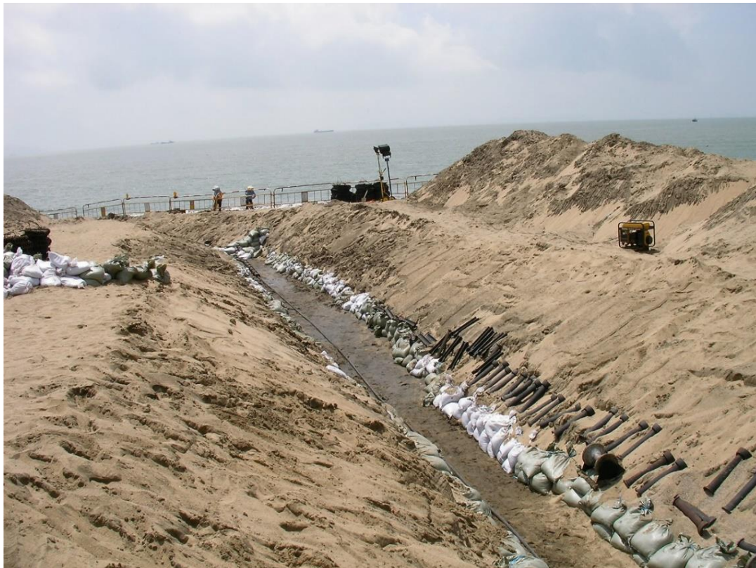
Figure 2-25 Example of Subsea Cable Installation by Trenching
