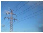
**Transmission lines:** In Zimbabwe it is proposed that the transmission lines will comprise of 2 x 70km 330kV lines, running in parallel, and sharing a common right-of-way, to the existing Hwange 330 kV substation. In Zambia, the line will comprise of 2 x 330kV transmission lines measuring 21km running
