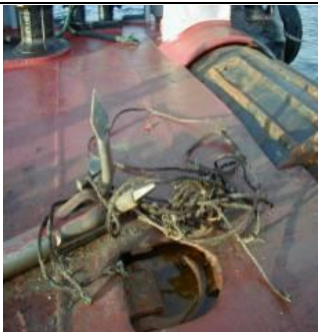
Figure 2.5 Equipment Used for the Pre-lay Grapple Run
