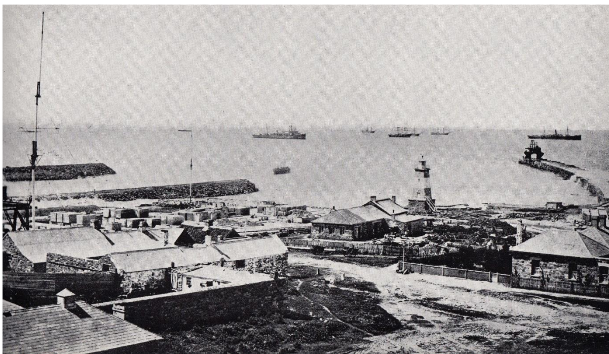
Plate 5: Entrance to the Buffalo River in 1882 from the west bank showing the Castle Point lighthouse between the breakwater (right) and the western training wall (centre left) (Source Denfield 1965: 16)
