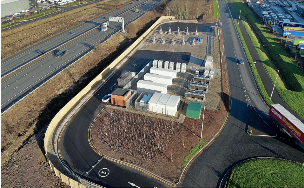
Figure 10: Example large scale CNG refuelling station operated by CNG Fuels in Warrington. Image courtesy of CNG Fuels
