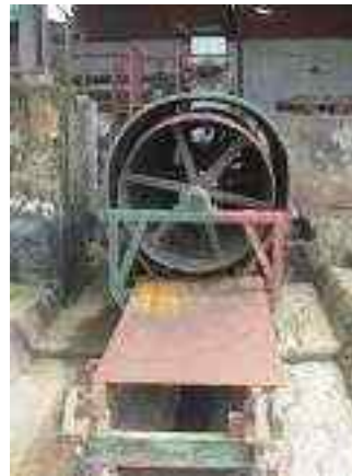
Screen cage (out of service)
