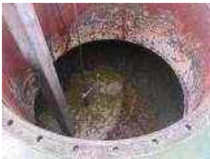
Collection tank (with fibrous mat)
