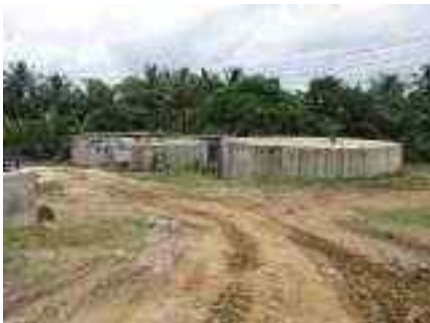
View of the two concrete digesters
