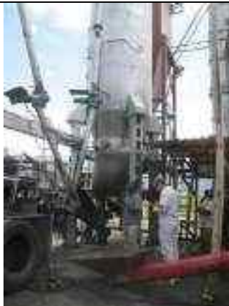
Reactor and ash removal
