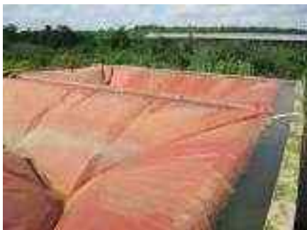
Digester bags (partly full)
