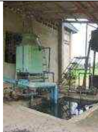
Water cooler and recirculation pond
