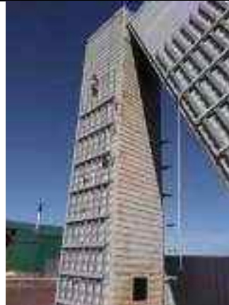
Reactor tanks being installed
