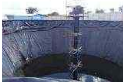
Second digester (under construction)
