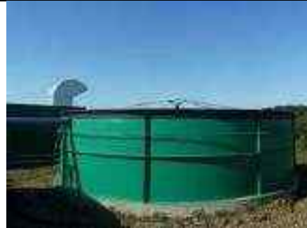
First digester tank
