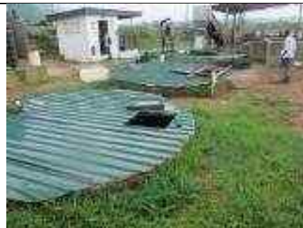
Liquid pre-mix tanks for latrine waste
