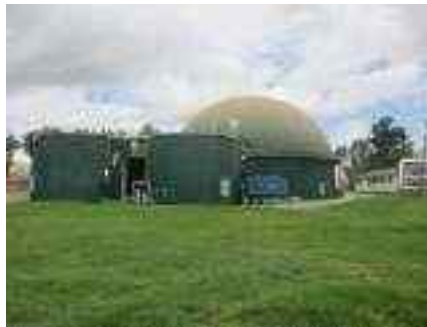
Site view with slurry storage tanks
