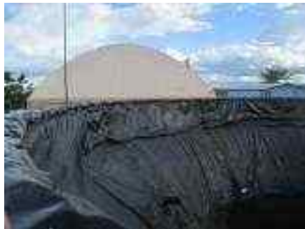
Completed digester (at rear)
