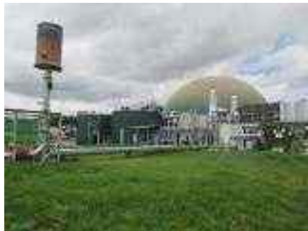
View of engine area
