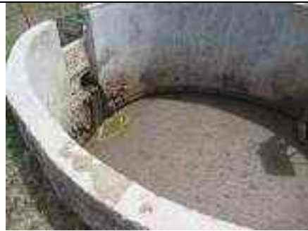
Slurry in pre-pit
