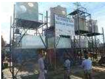
Integrated AD & water treatment plant
