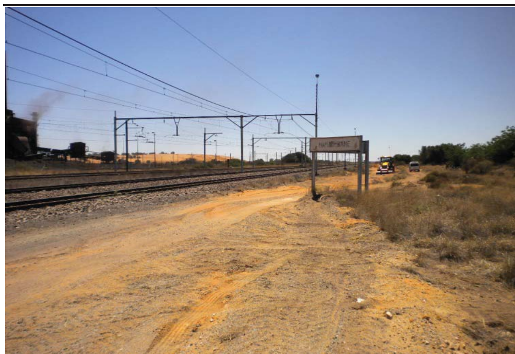
Figure 6.10 Railway Service Road
