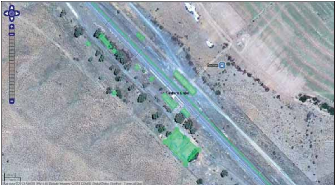
Figure 77: Drennan Station and various old railway structures (SAHRIS, 2013)
