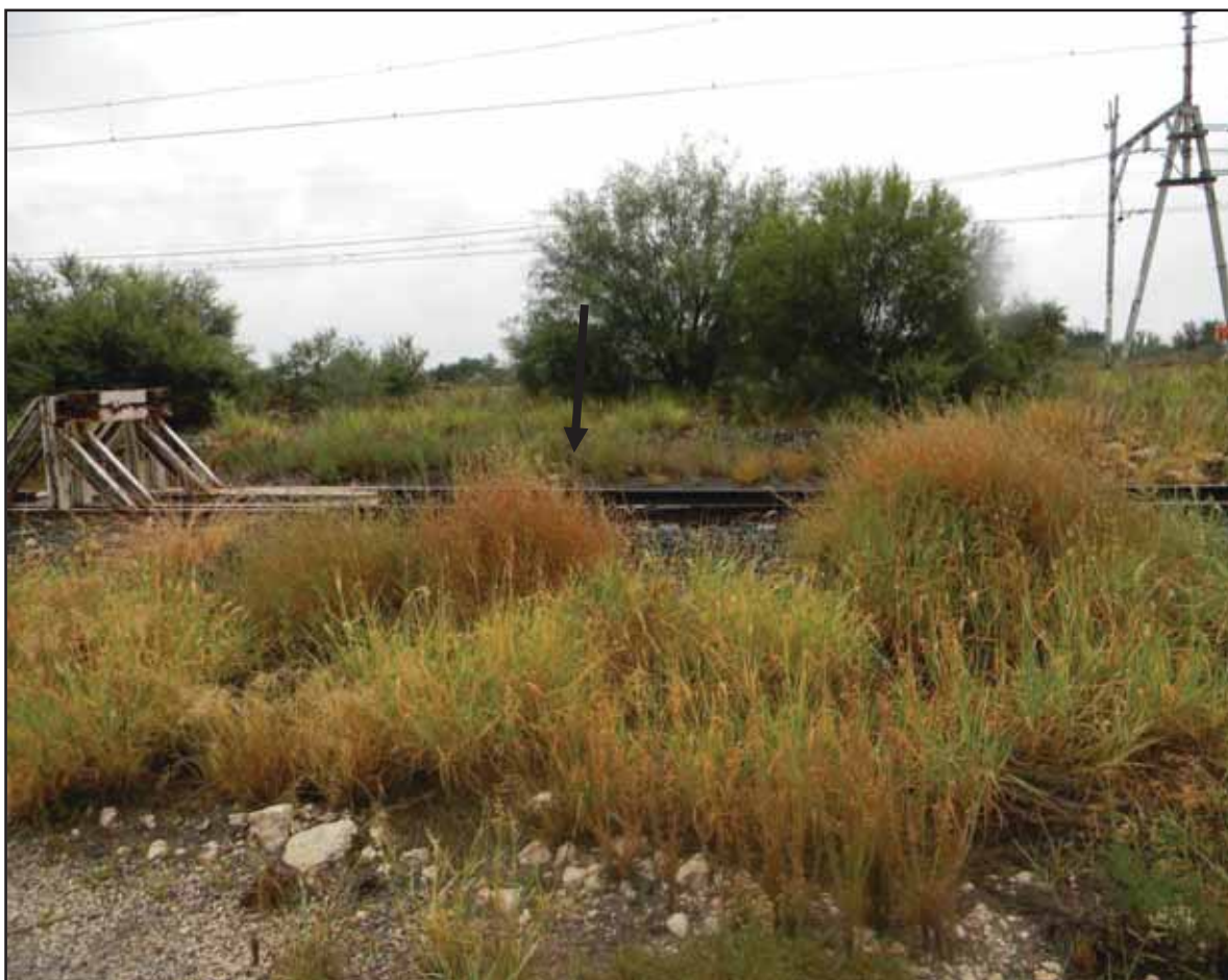
Figure 53: Old railway features at Ulco Station
