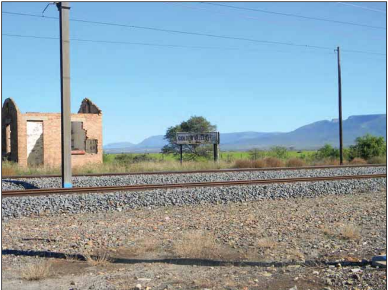
Figure 81: Golden Valley Station and historical structures
