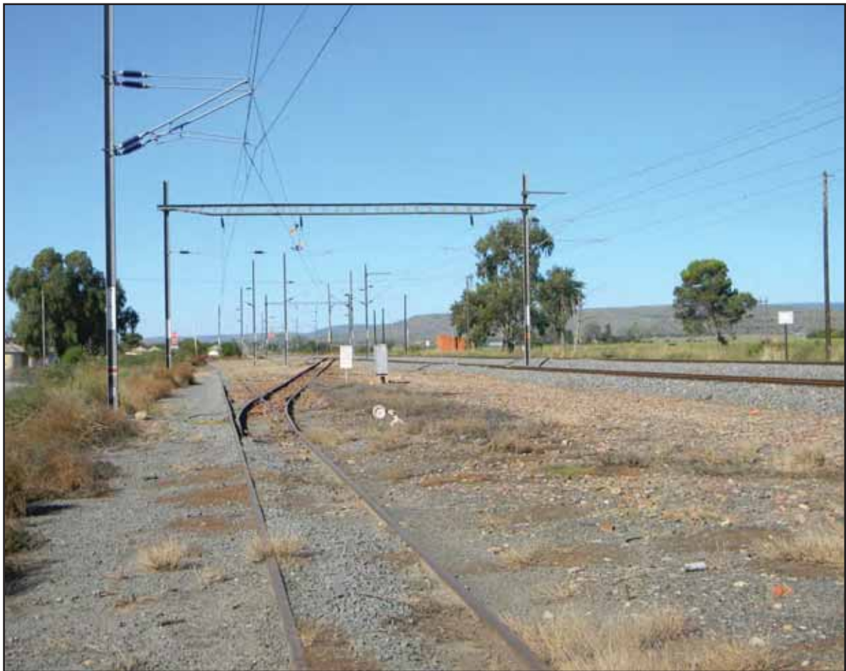
Figure 83: Railway infrastructure at Golden Valley Station
