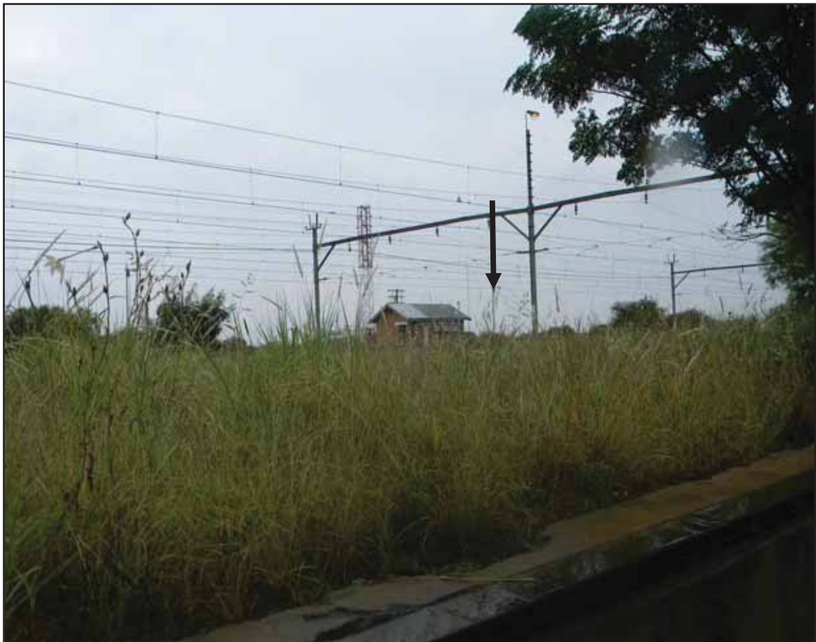
Figure 51: Railway buildings at Ulco Station
