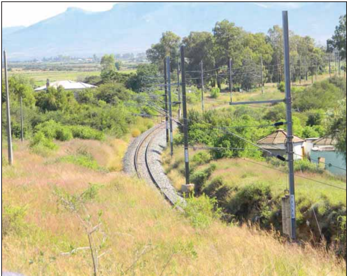
Figure 86: Railway line south of Golden Valley Station. Historical and temporary structures are situated alongside the existing railway line
