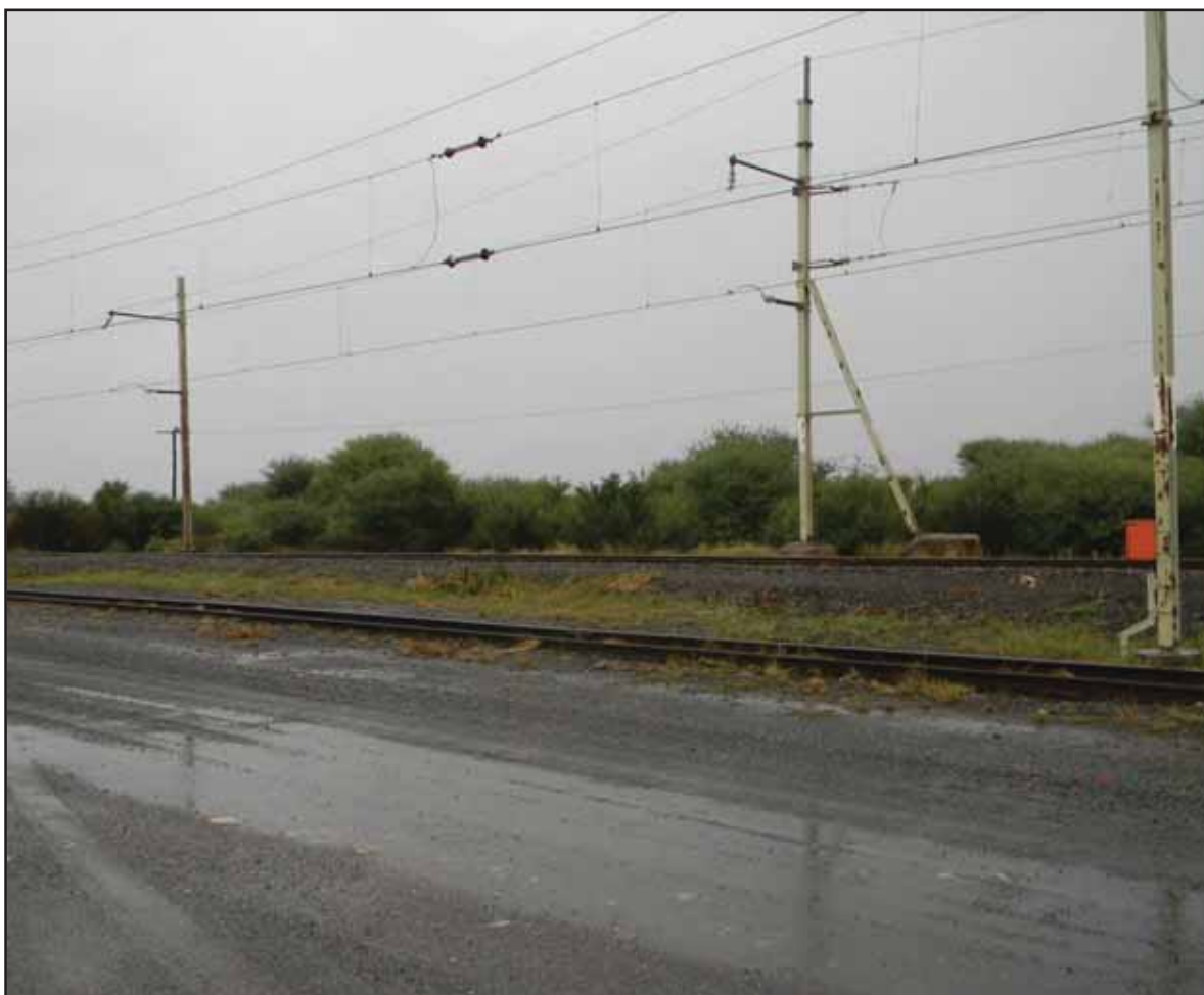
Figure 50: Railway reserve at Ulco Station
