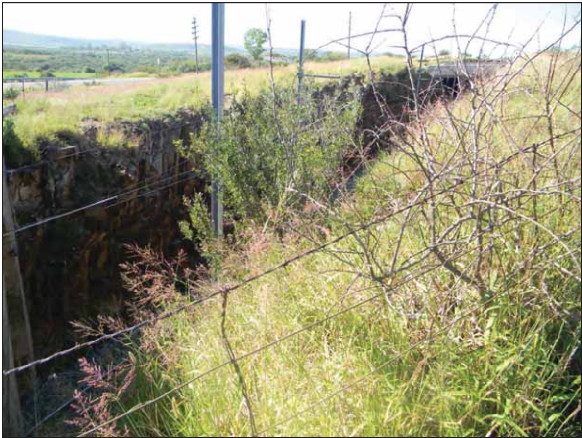
Figure 87: View of the railway line south of Golden Valley Station
