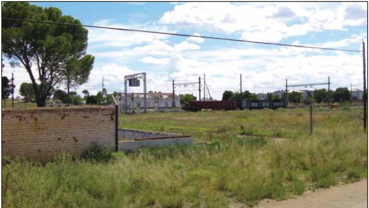
Figure 73: Rosmead historical structures and railway line
