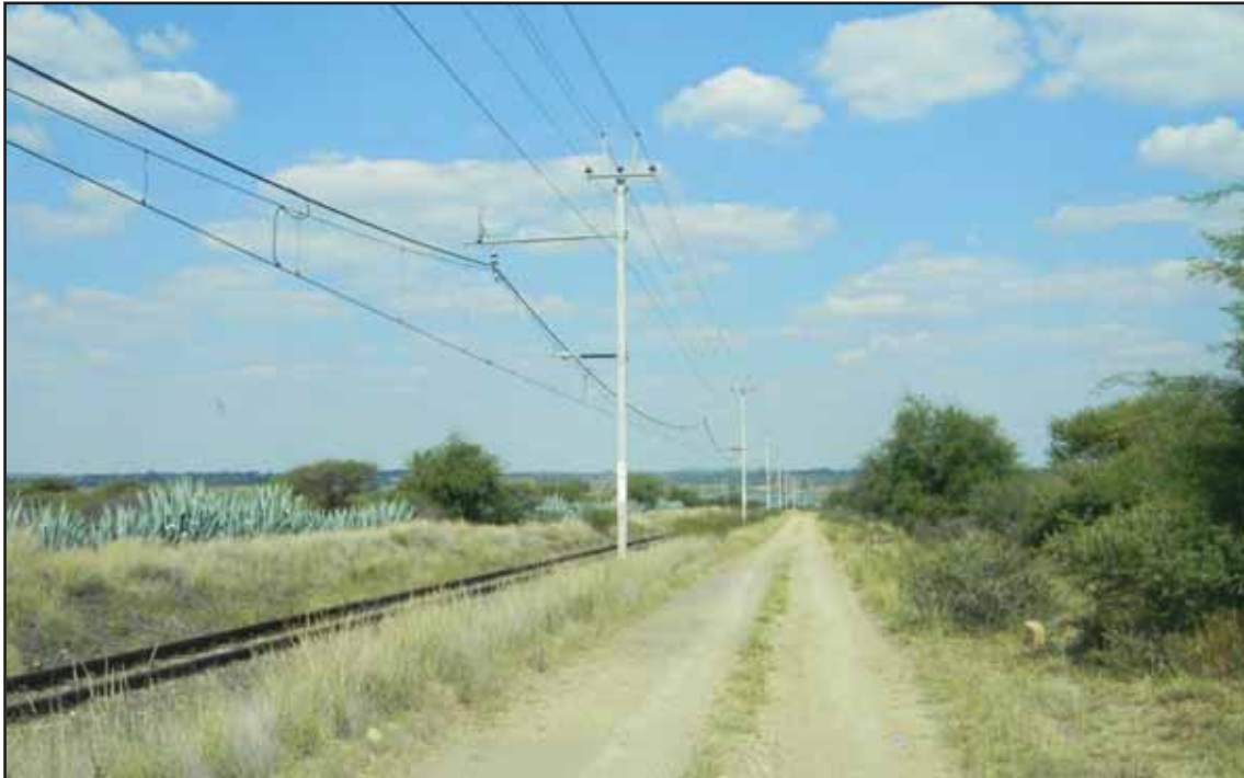
Figure 69: The railway reserve south of Fieldsview Station
