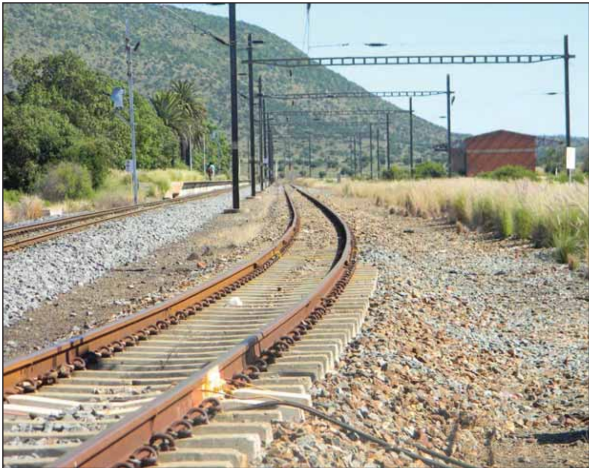
Figure 103: Railway tracks and structure situated at Kommadagga Station
