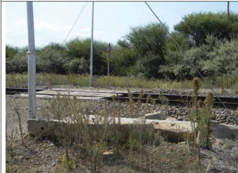
Example of a railway crossing at Winter's Rush
