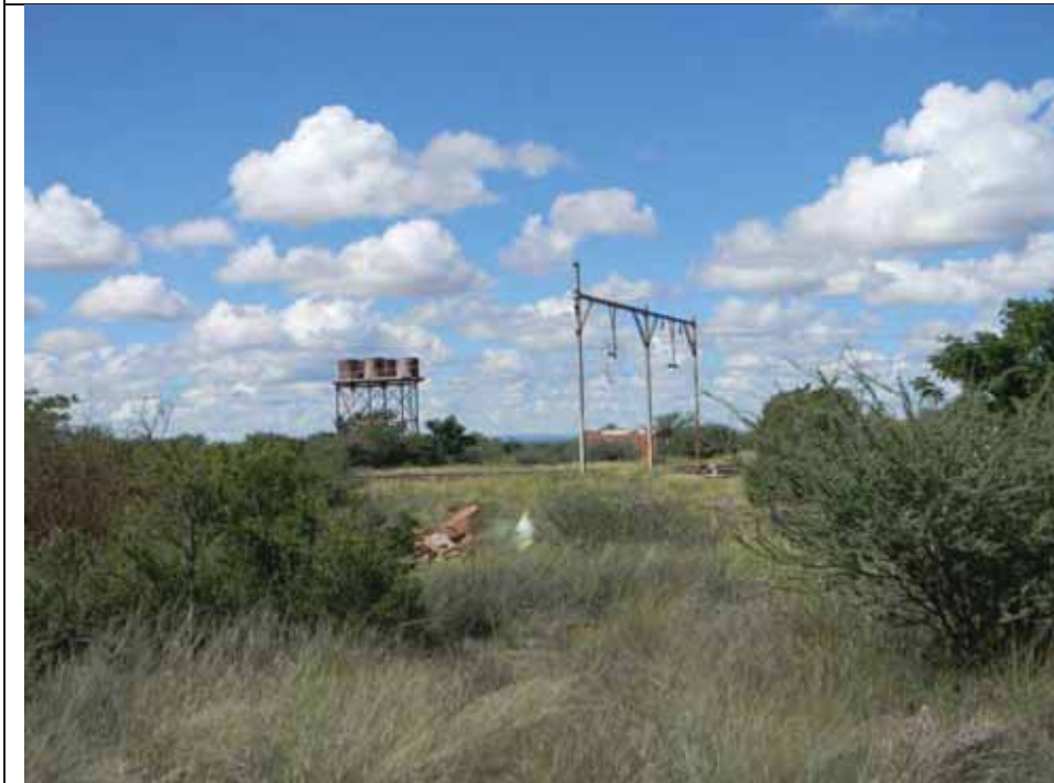
Railway line north of Sishen on the way to Hotazel
