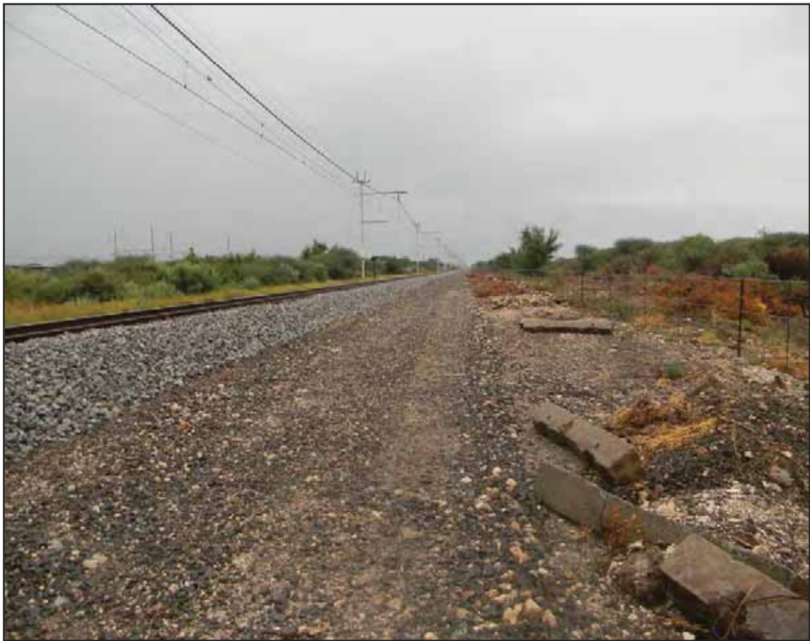
Figure 54: Area south of Ulco Station, towards Ghaap
