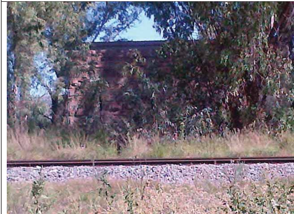
Blockhouse positioned next to the existing railway line at Visrivier area
