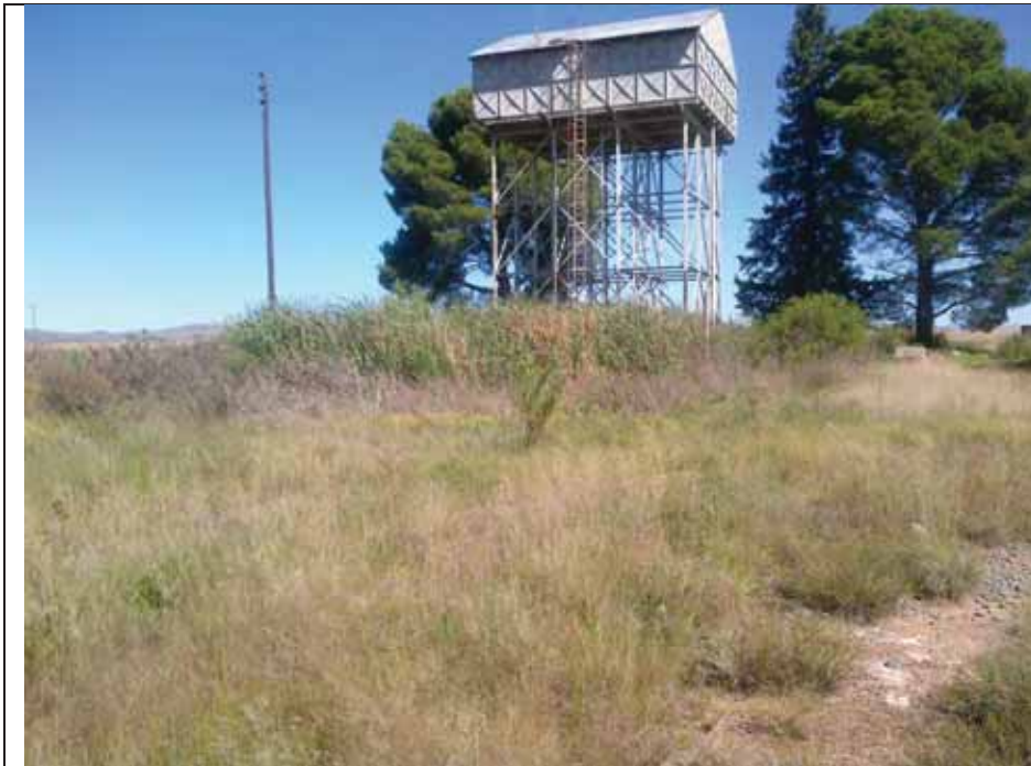
Historical water towers positioned next to the existing railway line at Visrivier area
