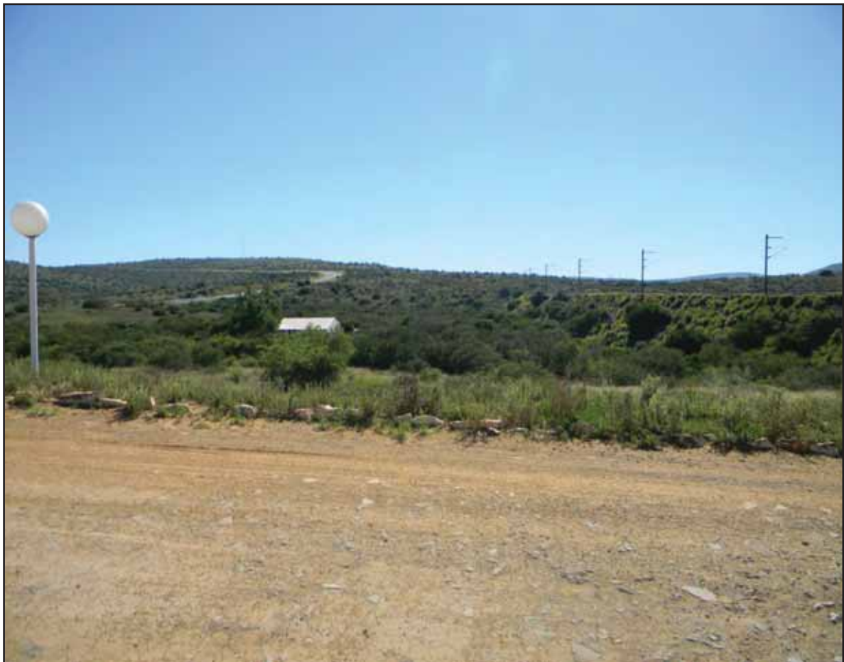
Figure 95: View of the railway line heading towards Kommadagga Station
