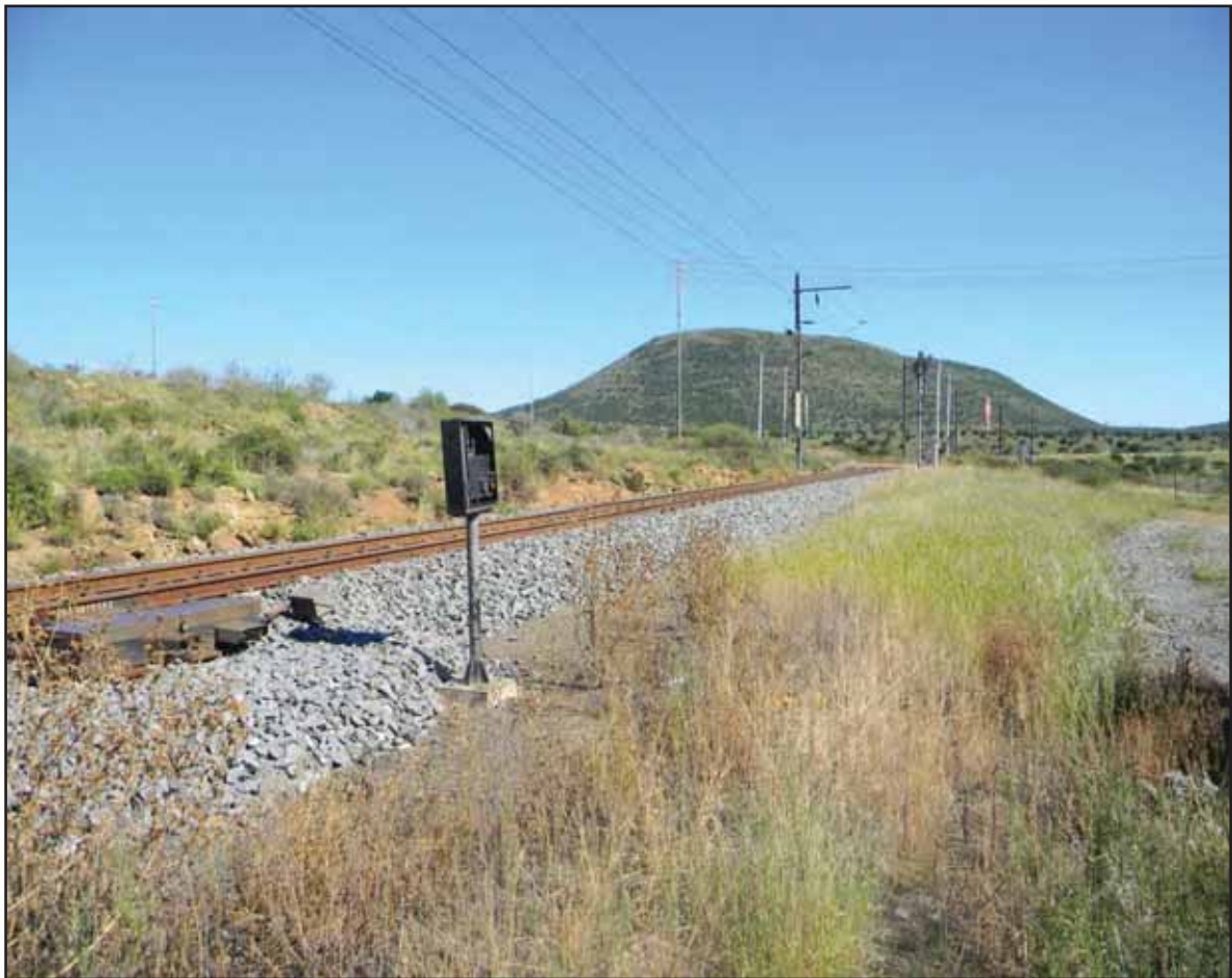
Figure 97: Station and line situated west from the existing railway line at Kommadagga Station
