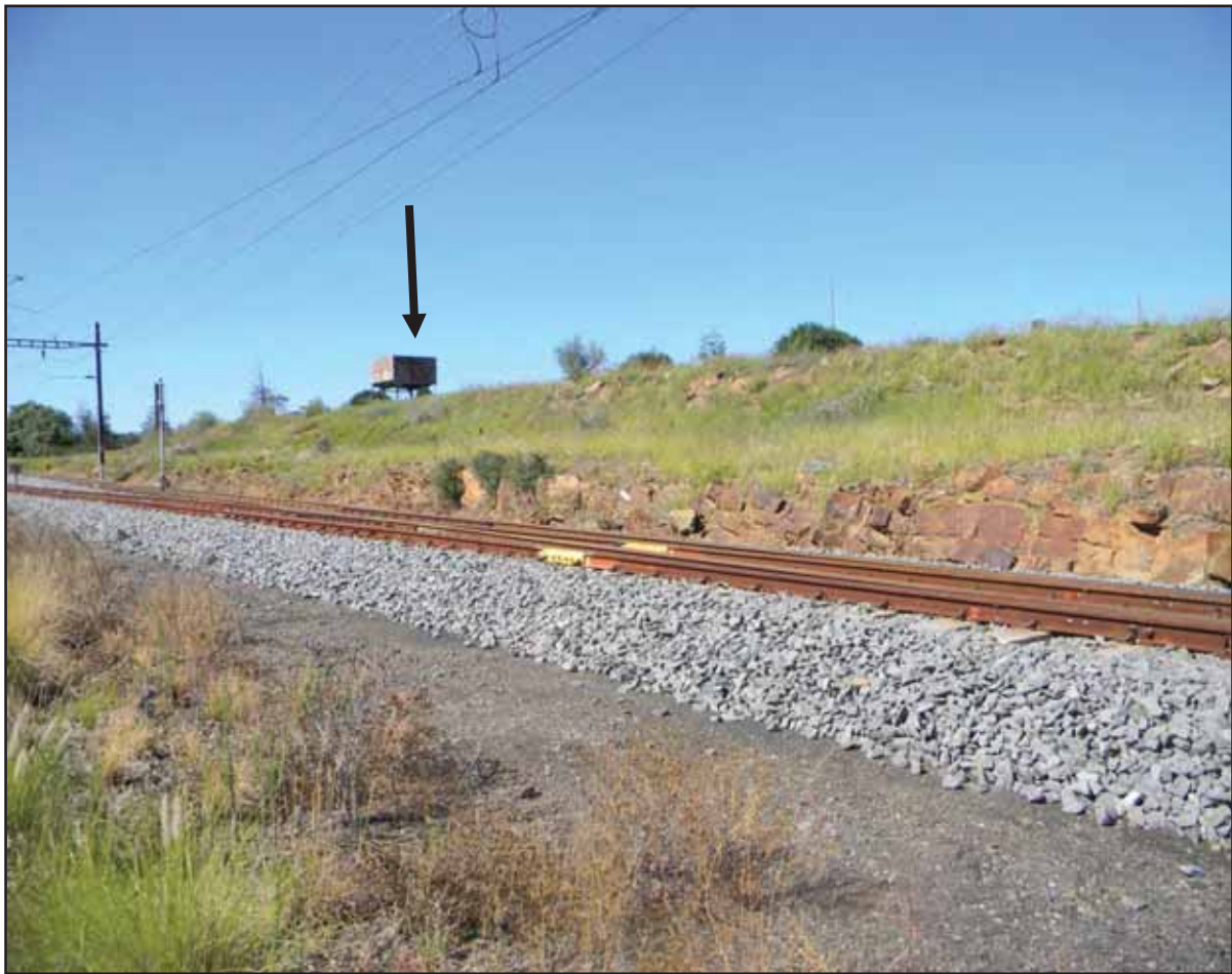
Figure 98: Historical water tank situated west of the existing railway line at Kommadagga Station The water tank will not be destroyed by the proposed development
