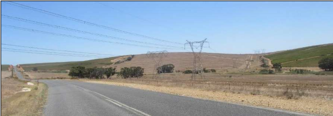
Photograph 3.2: 132 kV lines traversing the R 315 on Widschutsvlei Farm
