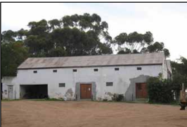
Figure 33: The east side of the barn.
