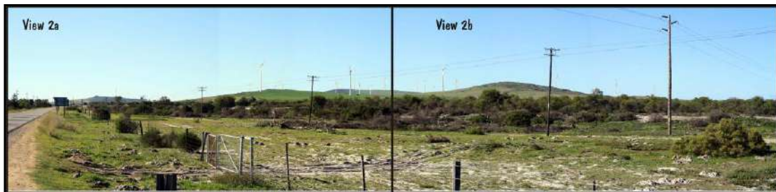
Figure 6b: Post-construction panoramic overview from Viewpoint 2 (showing photo sections).
