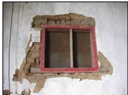
Figure 36: An opening inside the western half of the barn in the central wall.
