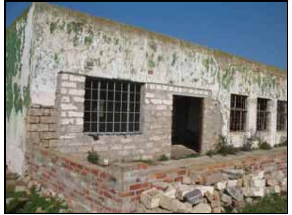
Figure 55: The old school building.
