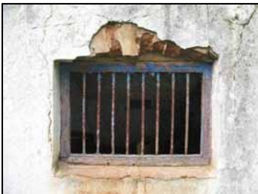
Figure 35: An external opening on the west side of the barn.
