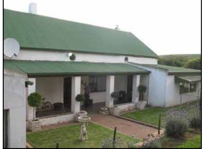
Figure 58: The eastern side of the Rheboksfontein main house.
