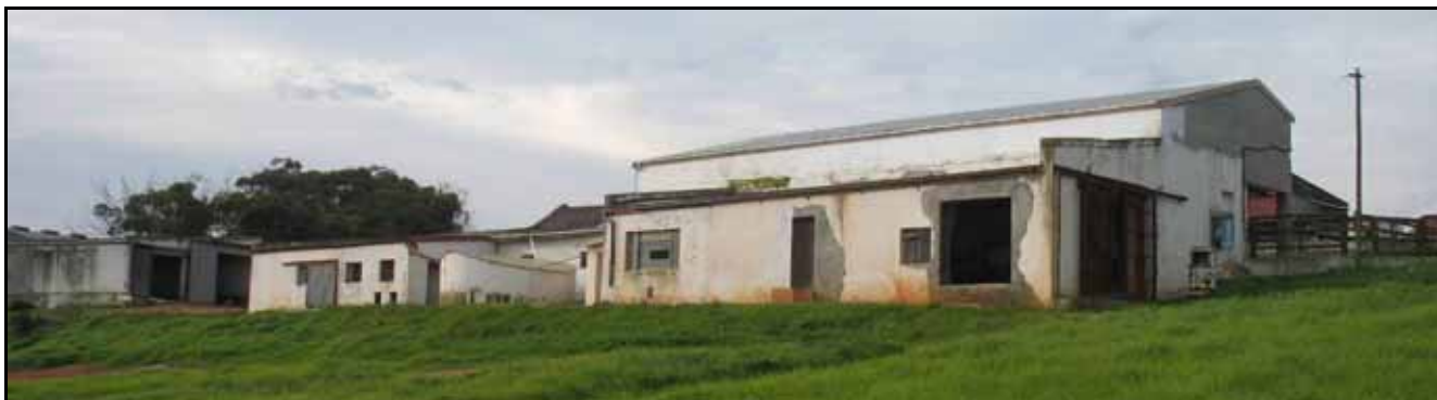
Figure 62: View of the western side of the dairy showing the extensive alterations.
