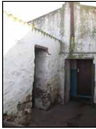
Figure 50: An addition to the dairy displaying stone walls up to door-height.
