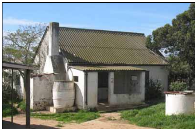
Figure 68: The west face of the corrugated iron cottage.
