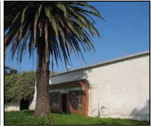
Figure 51: Another structure with modern alterations.
