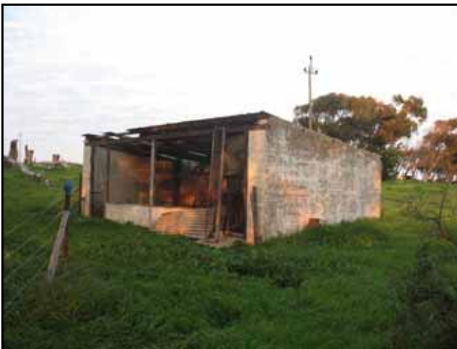
Figure 44: A shed built with decorative breeze blocks suggesting 1930s or 1940s. Its roof has been changed more recently.
