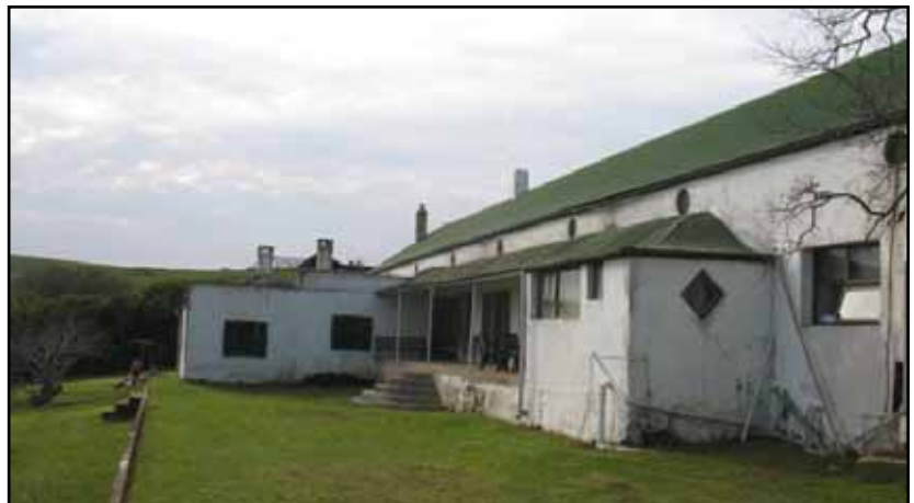
Figure 60: The front, west-facing façade and porch with its curved corrugated iron roof.
