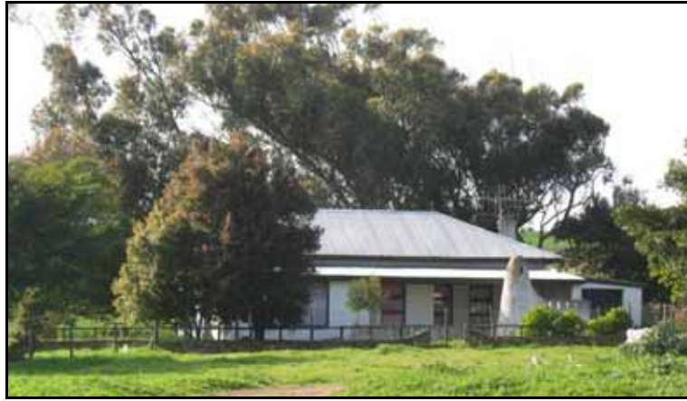
Figure 41: House east of the main farm house that has had extensive modification.
