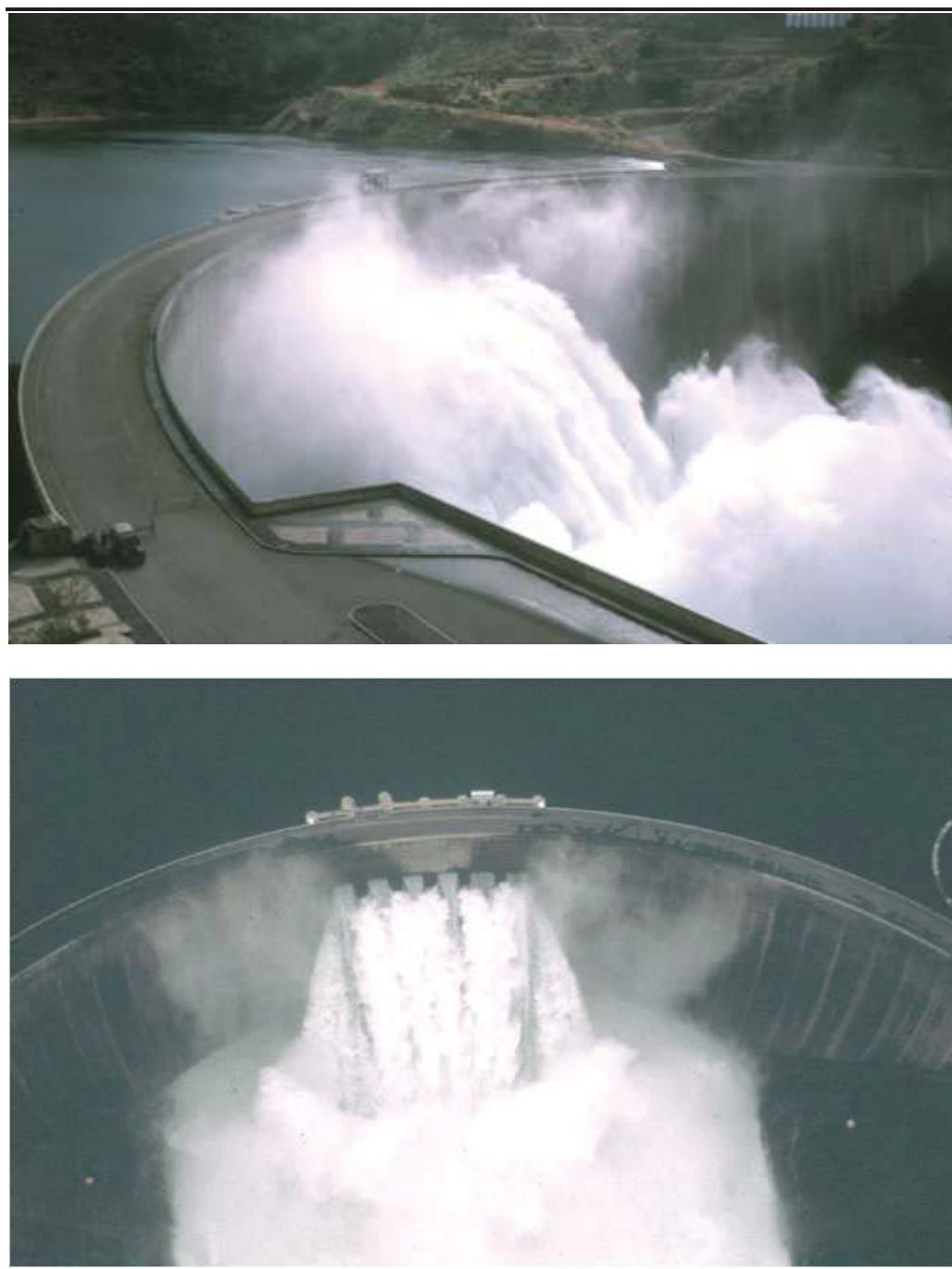
Figure 2.4 All Six Sluice Gates Open during a Test Spillage (1966)
