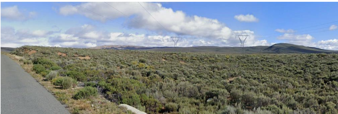
FIGURE 5-26: EXISTING POWER LINES WITHIN THE STUDY AREA
