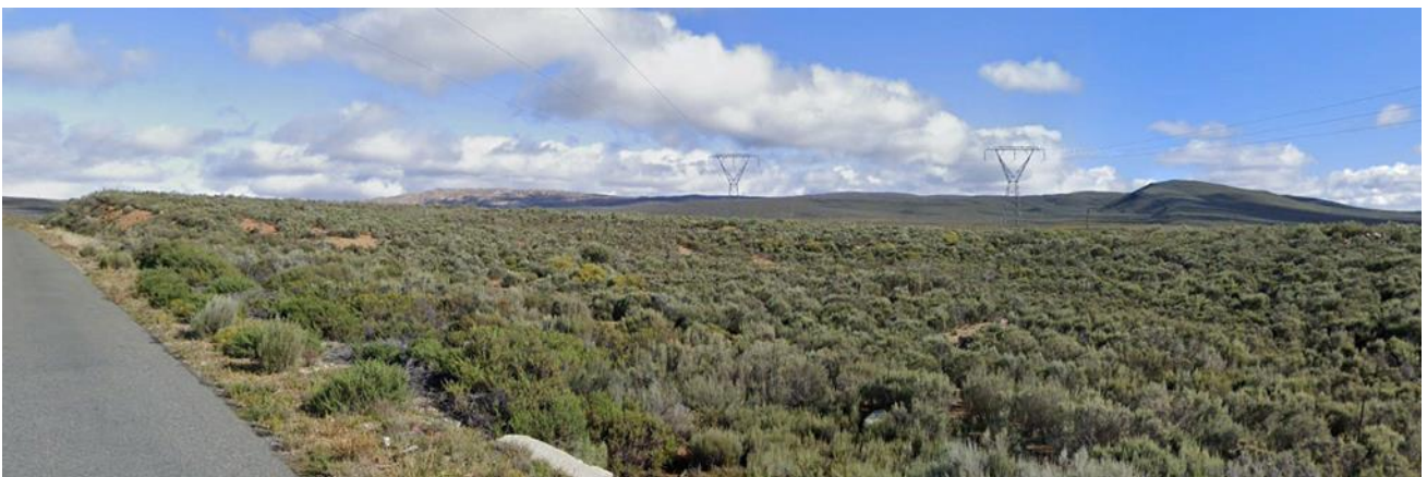
Figure 7: Existing power lines within the study area
