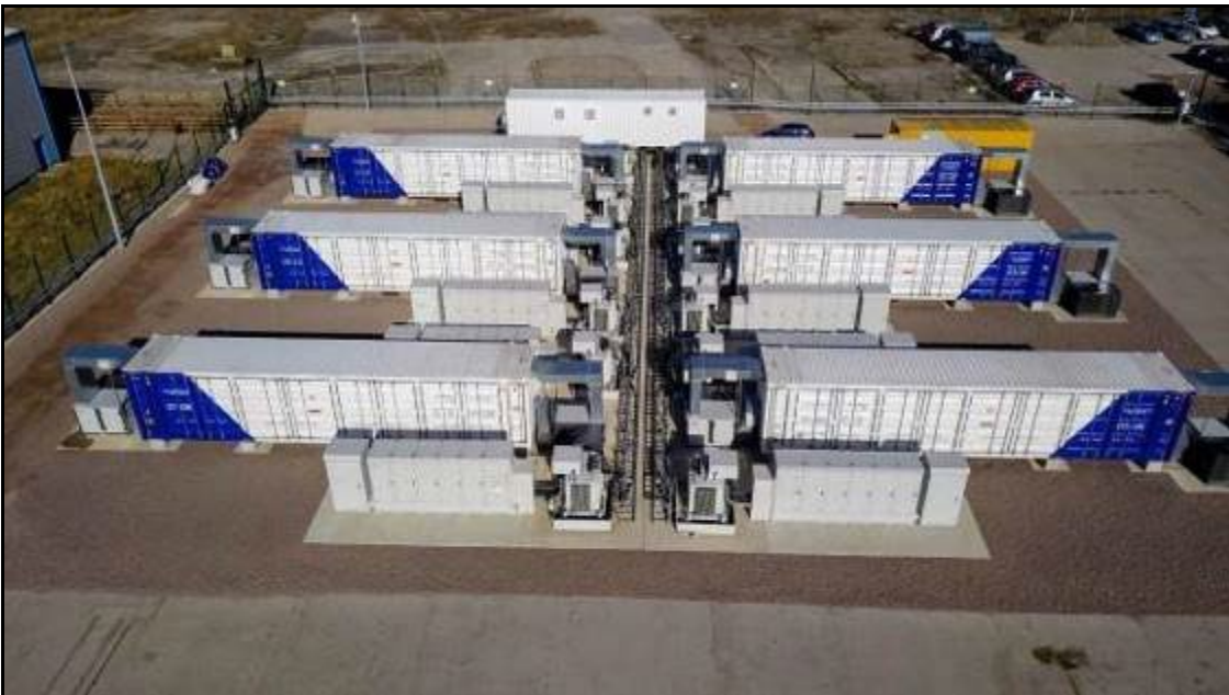
Photograph 1.2: Example of BESS located in storage containers
