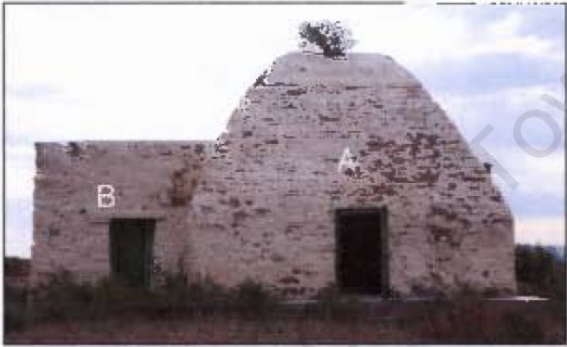
Figure 37: The corbelled house at Vaalhoek. Source: Kramer (2012: fig. 6-34).
