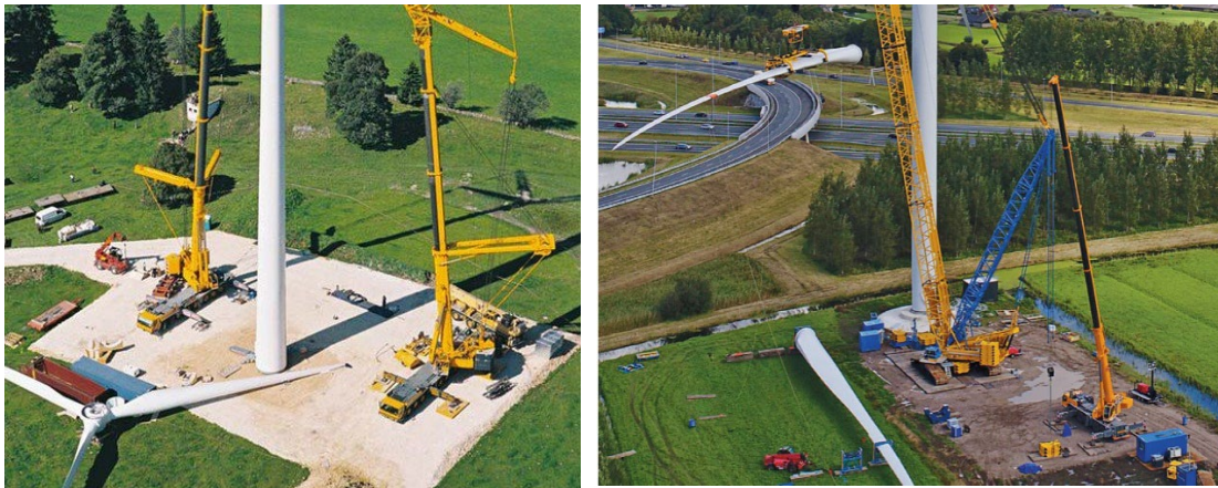
Plate 9-4: Illustration of a typical Turbine Hardstand and Laydown Area
