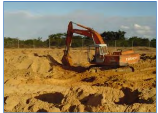
Using mixed-bury-cover (MBC) to dispose of drilling waste at Inhassoro well pads
