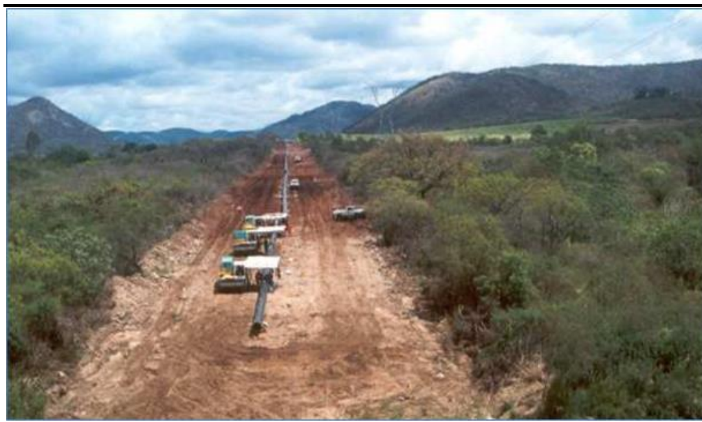
Figure 2.5 Example of the Construction of a Pipeline and Associated Right of Way
