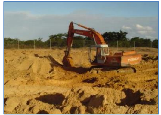
Using mixed-bury-cover (MBC) to dispose of drilling waste at Inhassoro well pads
