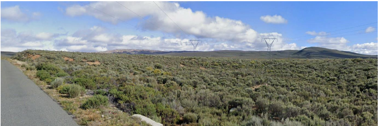
FIGURE 5-29 EXISTING POWER LINES TRAVERSING THE PROPOSED HUGO SITE
